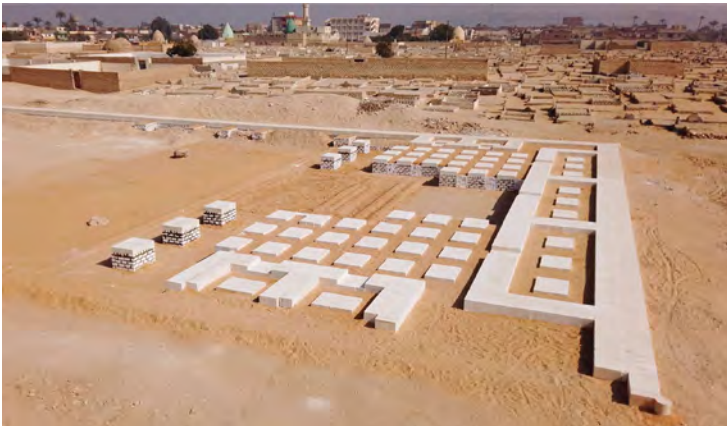
A view toward the north showing the ground plan and offering table reconstruction underway in the sixth court of the Long Temple
